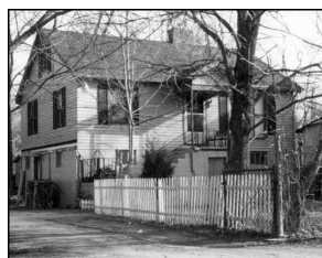
1536 East 73rd Street The Picket fence was added later.
